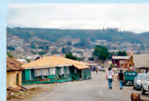
Pelluhue after the earthquake.
