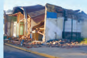
Earthquake damage in Angol.
